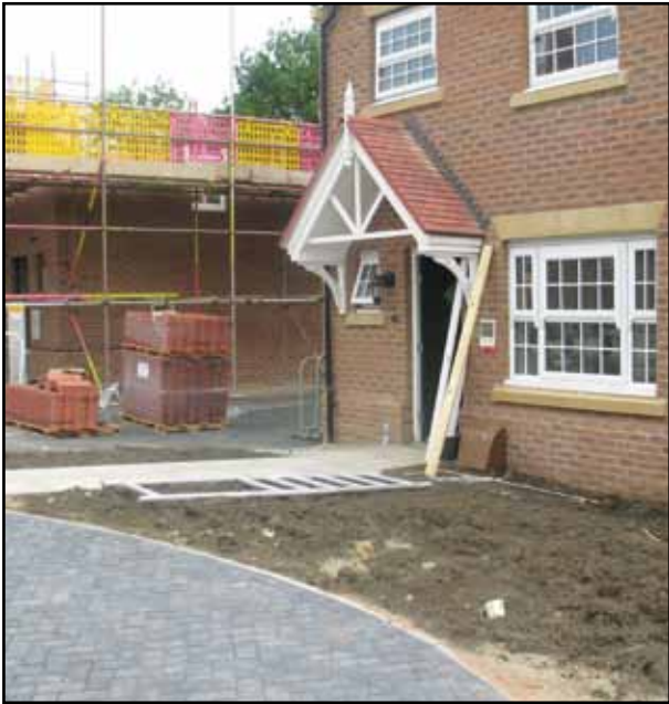
Construction at the Oaklands, in Easingwold
