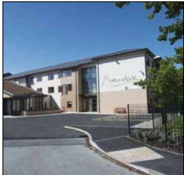
Extra Care Housing - Rivendale in Northallerton
